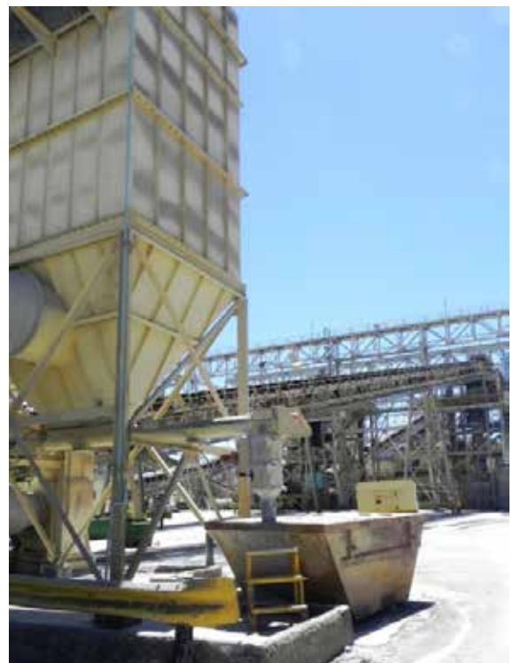
Figure 19: Fine crushing dust collection system
